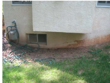
Re-grading Needed
