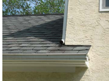
Downspout Emptying on Roof (typical)
